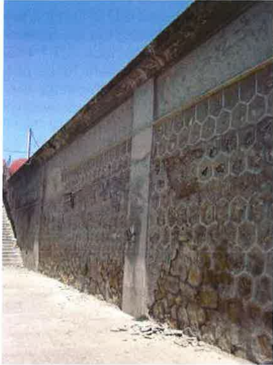
Figure 3.1. Masonry wall along Guadalentín river bank passing through Lorca, used as a marker.
