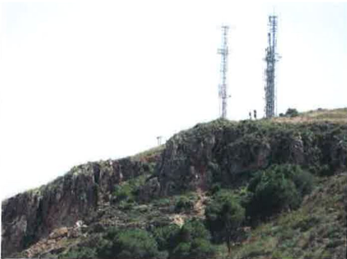
Figure 4.5: Communications towers founded on a hill situated in front of the westernmost end of Lorca's castle cliff. Two recent instabilities are shown, which are attributed to the 11 May earthquakes.
