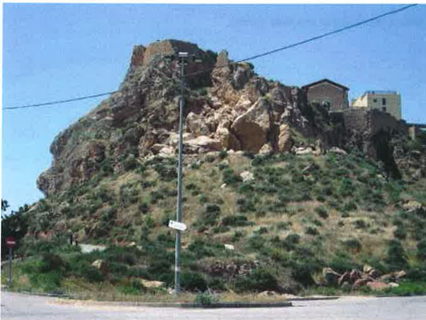
Figure 4.2.1a: Partial collapse of the easternmost point of Lorca's castle cliff. A detached rock-block produced damage in a near house (see Fig. 4.2.1c). Picture on right corresponds to the same place few years back (taken from the IGME seismic hazard study of Lorca, 1992).
