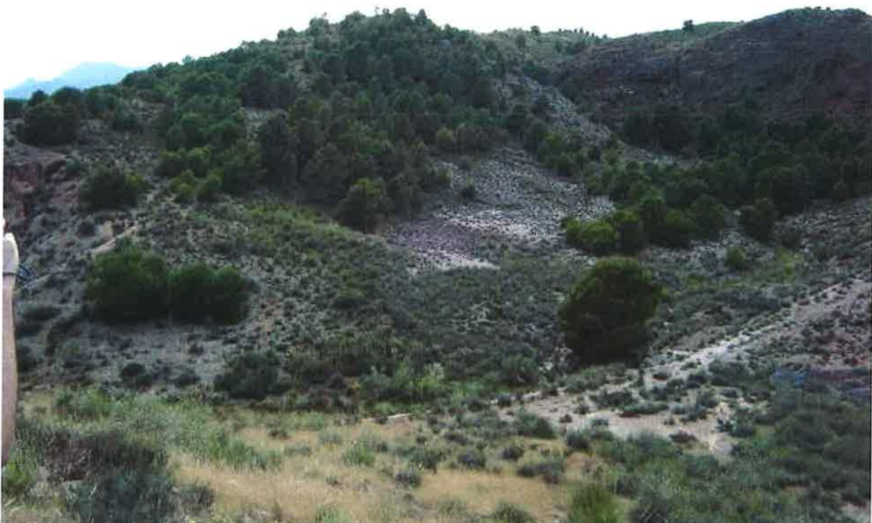
Figure 3.3. Concrete fence basement used as a marker to look for deformation along the fault line of the FAM.
