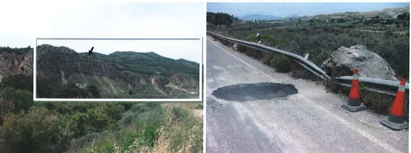
Figure 4.4.1b: Continuation of the Pantano de Puentes road towards the west. Along this road many instabilities were identified, although of a small size in general. Particularly remarkable are the rock blocks fallen from the ridge controlled by Las Viñas Fault (marked with an arrow). Picture on right shows a close-up of the damage produced by one of this rock blocks.
