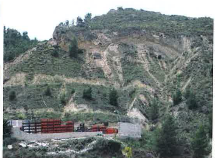
Figure 4.6: View of the slope enclosing a butane-gas storage site on the Pantano de Puentes road. No slope instabilities that could be attributed to the earthquakes were identified here, although the collapse of the concrete-brick wall is attributed to them.
