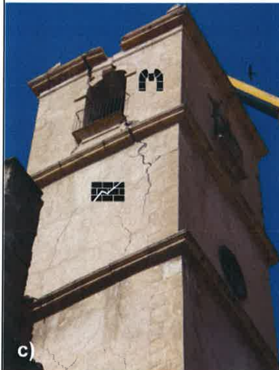
Figure 5.6: Damage in the San Francisco's Church.
