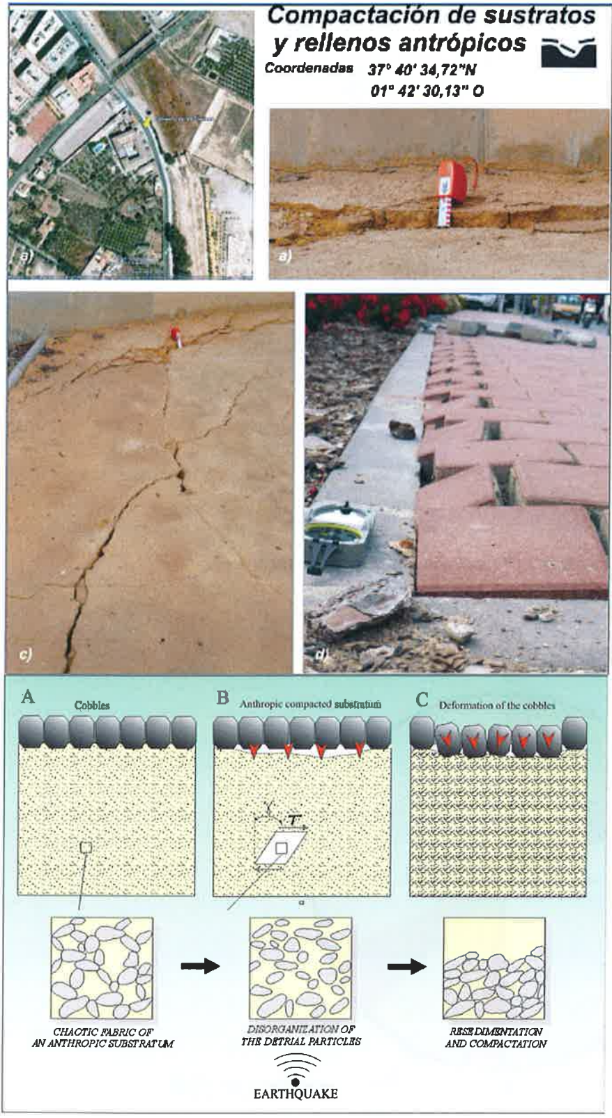
Figure 5.9: Anthropically compacted substratum by seismic shock related to the Clarisas's Convent. New EAE structure.
