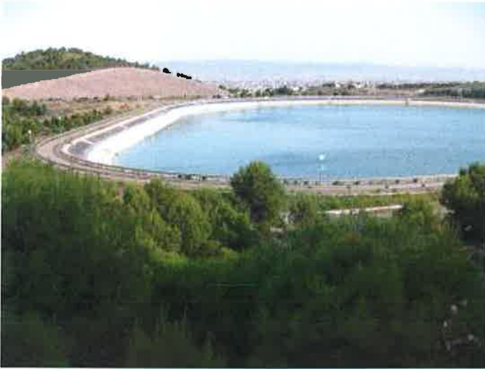
Figure 4.7: Irrigation pool situated nearby the epicentres of the 11 May earthquakes. Neither damage was observed in this area, nor instabilities on the talus on the background.
